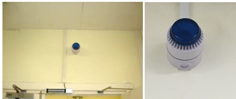
Figure 3: Visual and auditory beacon for O2 below 18%
